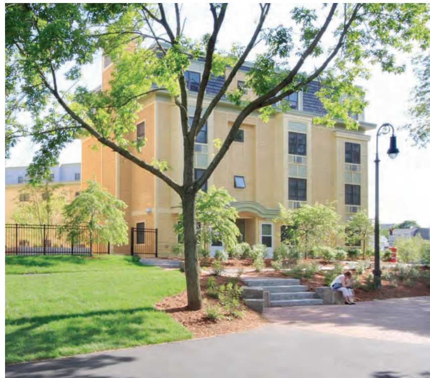
Trolley Square in Cambridge, Massachusetts. Green homes open onto Cambridge Linear Park, a bicycle and walking path.
